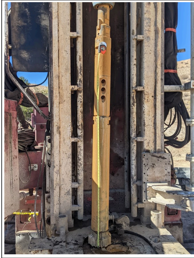
11. 2/7/2021: Major Drilling hammer assembly (view to west)
