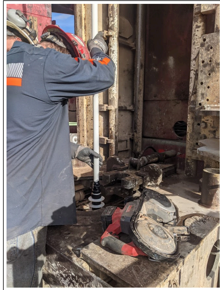
24. 2/3/2021: Crew deploying PVC swab to agitate well during development at monitor well 286-2021-01
