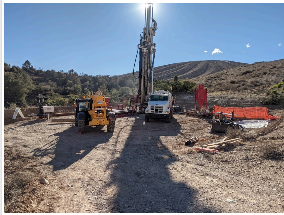
7. 2/4/2021: Major Drilling rig set up at 166-2021-01 location (view to west)
