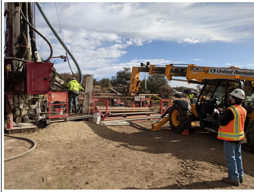
13. 1/19/2021: Freeport safety representative reviews safe pipe handling procedures (view to east)
