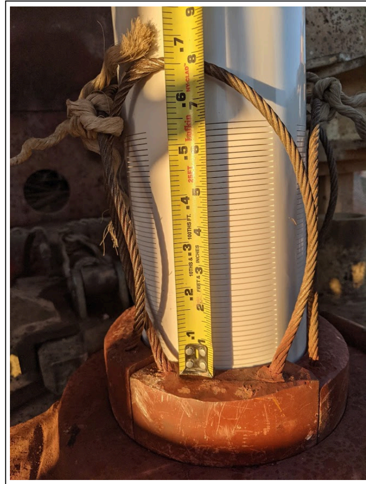
18. 2/13/2021: Measurement of 0.020-slot 5-inch-diameter SCH 80 PVC slotted screen
