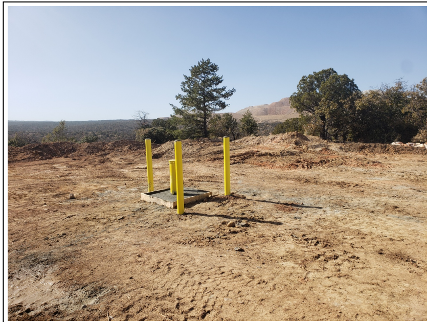
26. 2/28/2021: Example of surface completion at monitor well 396-2021-02 consisting of concrete filled bollards, locking well cap and concrete well pad (view to northwest)
