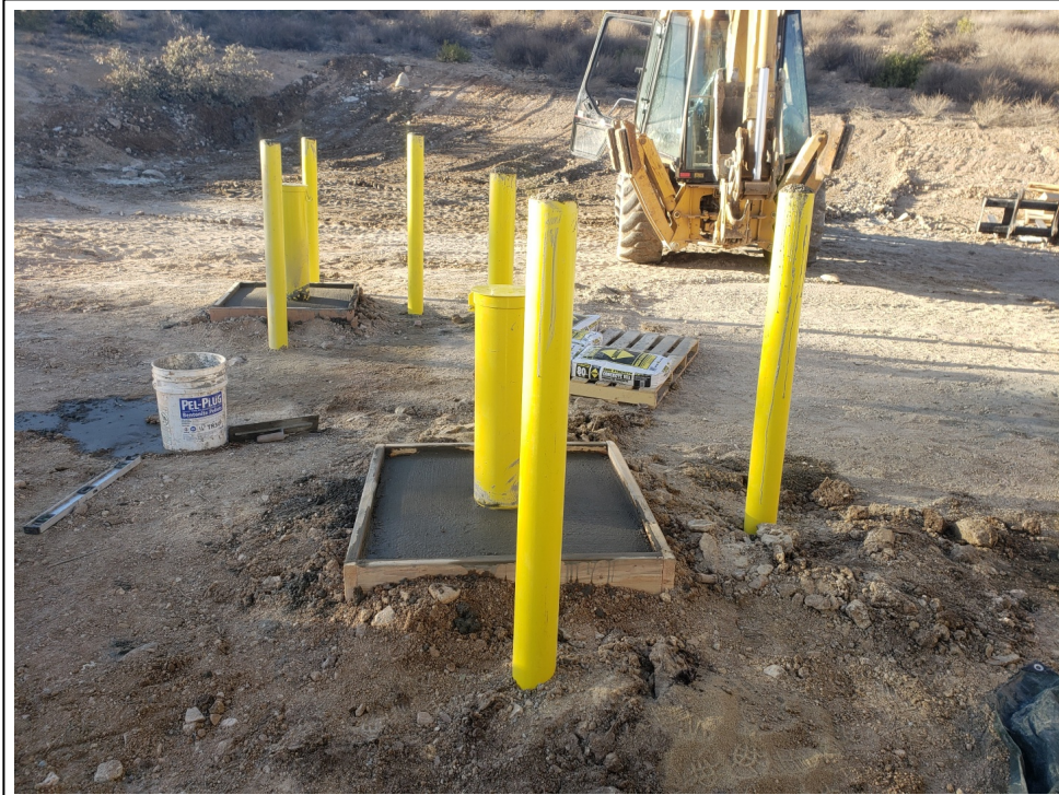
27. 3/4/2021: Surface completions at monitor wells 166-2021-01 (right) and 166-2021-02 (left) (view to north)
