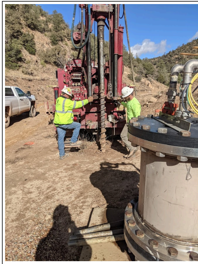
2. 12/10/2020: Enviro-Drill advancing borehole 166-2020-01 using hollow-stem auger method (view to north)
