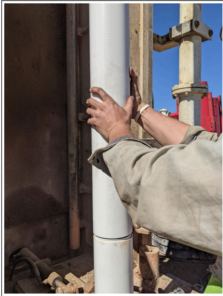
19. 2/24/2021: Installation of 5-inch-diameter SCH 80 PVC slotted screen
