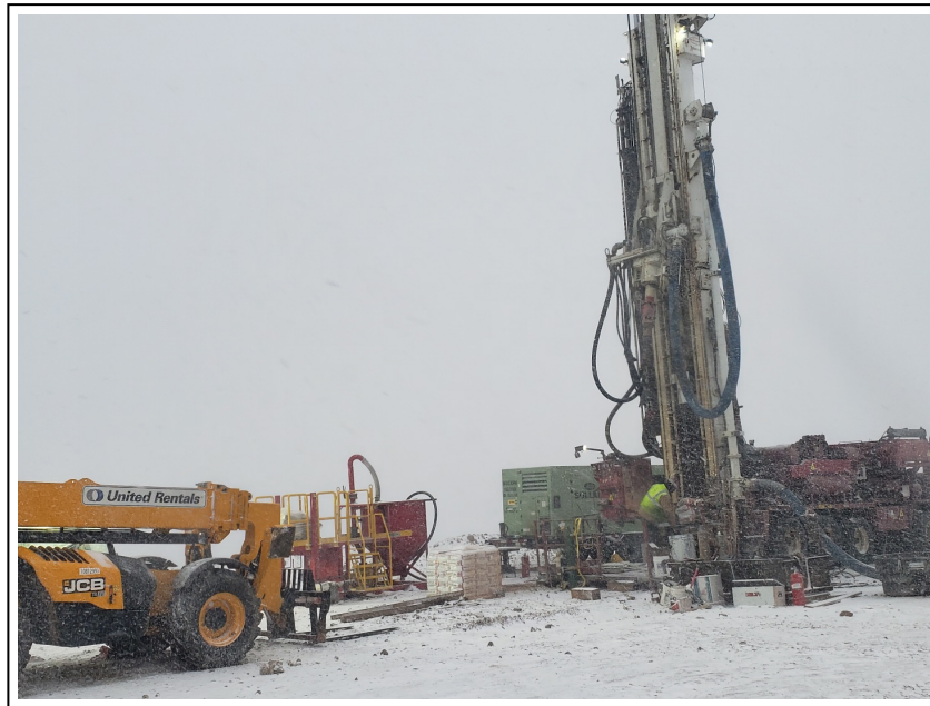
6. 2/14/2021: Major Drilling advancing GLD-4A replacement well 455-2021-01 in snow (view to west)
