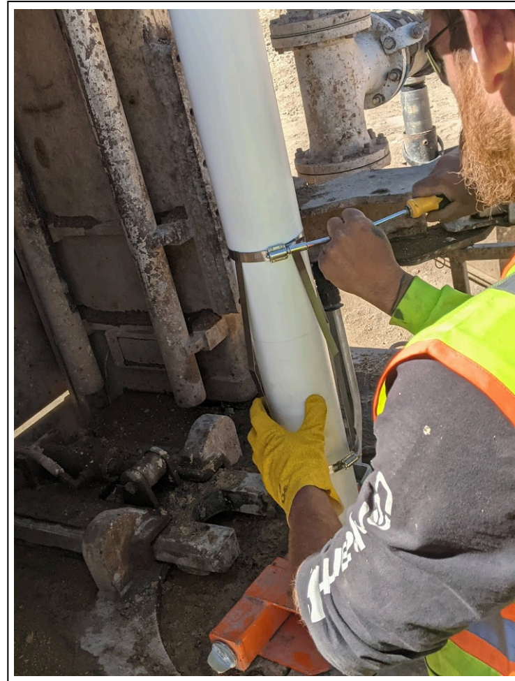
20. 2/24/2021: Centralizer being installed above screen interval at monitor well 396-2021-02
