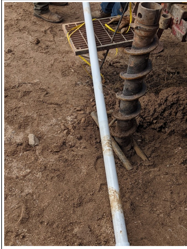
3. 12/10/2020: 166-01-2020 2-inch SCH 40 PVC screen and well assembly
