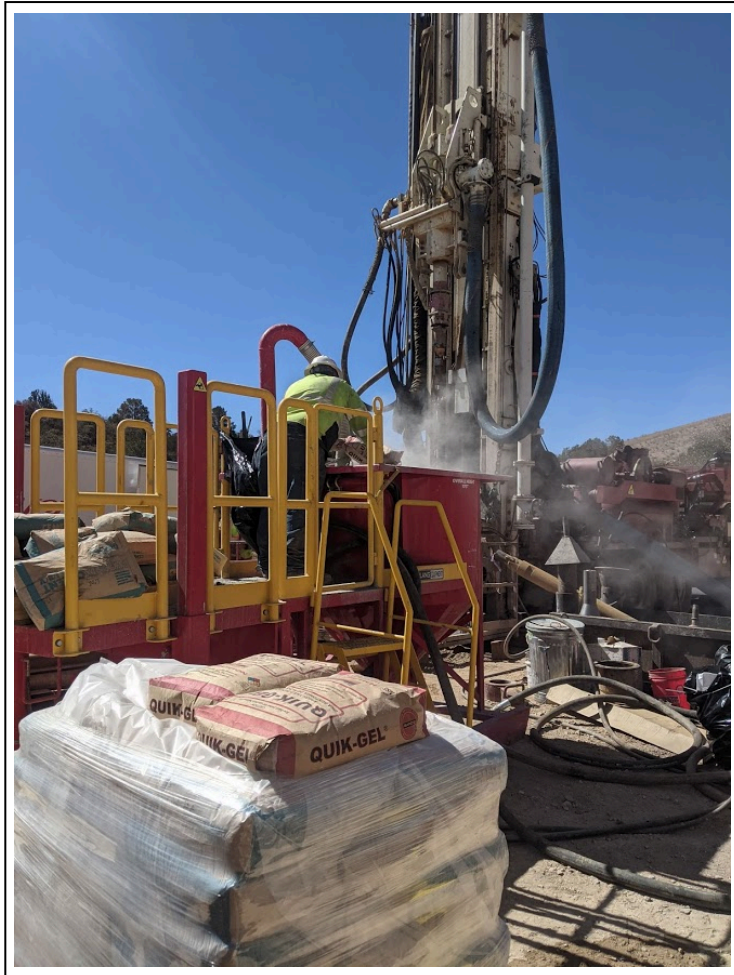
23. 3/2/2021: Major crew mixing 5% bentonite cement grout (view to southwest)
